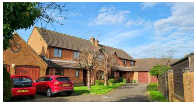
Figure 49: Typical style of semi-detached houses
