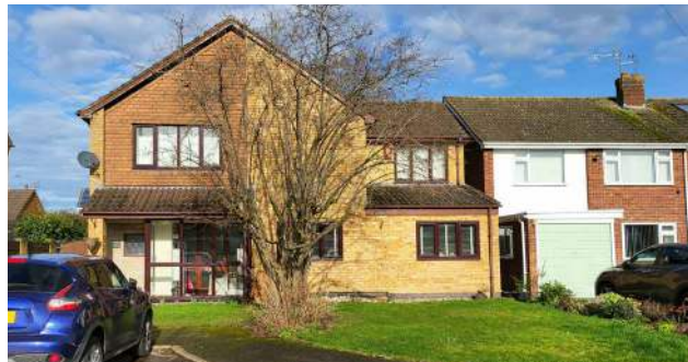
Figure 48: Typical style of detached houses
