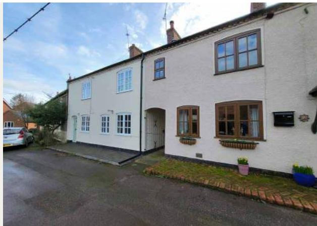
Figure 28: White rendered buildings along Little London Lane
