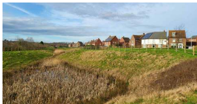
Figure 22: An attenuation pond which forms part of the SuDS strategy for part of a new residential development within the west of the neighbourhood area.
