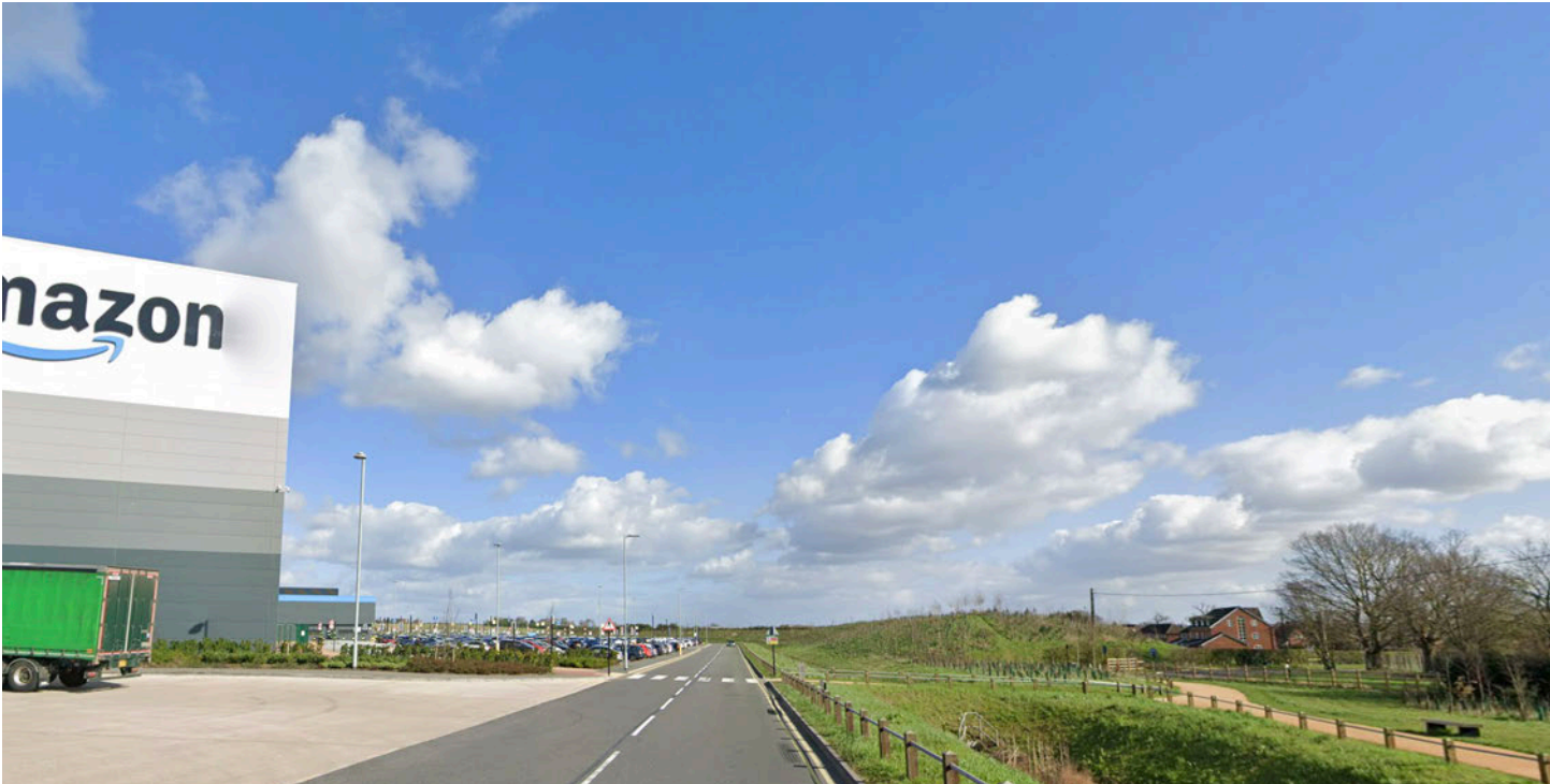
Green buffer with informal path and amenity adjacent to building , Peddimore industrial Estate, Sutton Coldfield, Birmingham
