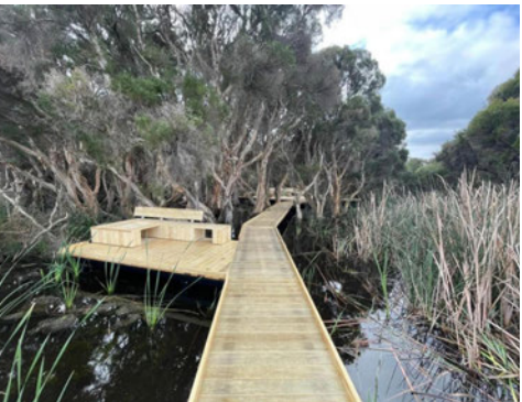
Timber wetland boardwalk
