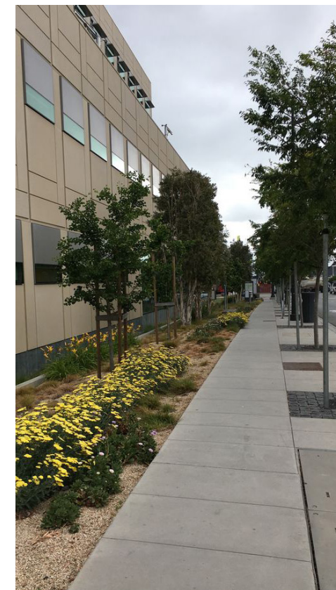
Urban bioswale/ rain garden running alongside a commercial building
