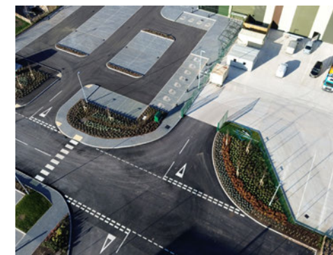
HGV and operational areas softened by integrated planting
