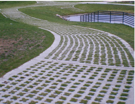
Grass-concrete / reinforced grass
