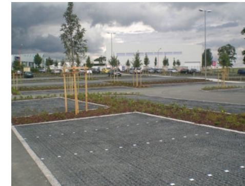
Permeable surface treatment within planted parking areas
