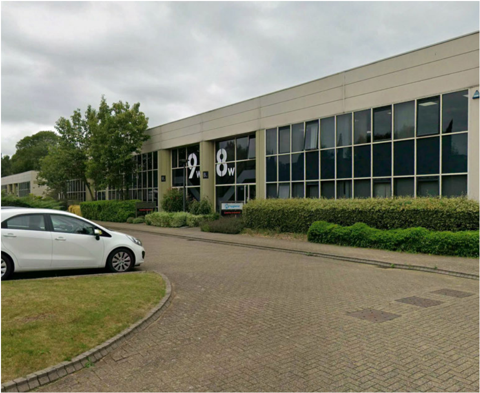
Wall and glass creates visual break, Croxley Business Park, Watford
