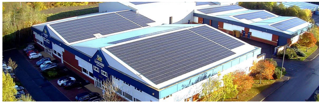
Solar PV roof, East Kilbride, Scotland
