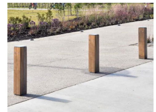
Timber bollards defining a route edge
