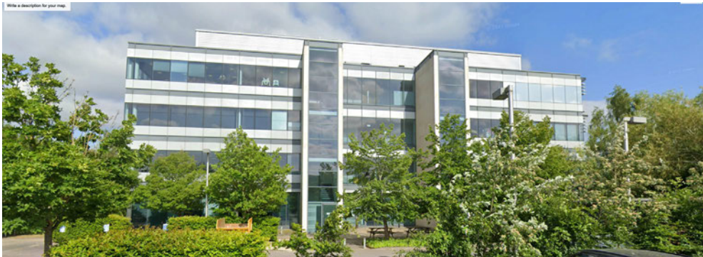
Office element, Green Park, Reading
