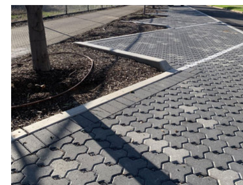
Permeable paving
