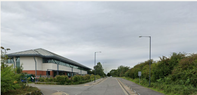
Rugby Free Primary School as viewed from the public bridleway near the western site boundary
