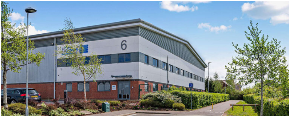
Contrasting cladding colour, Gateway 12 Business Park, Gloucester
