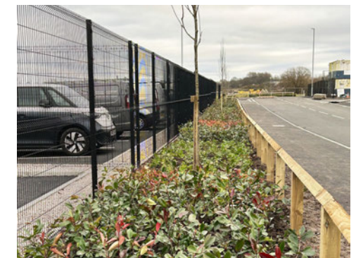
Security fencing set behind a substantial planted edge
