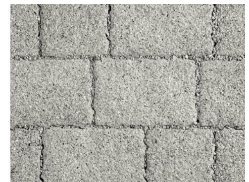
Permeable block paving
