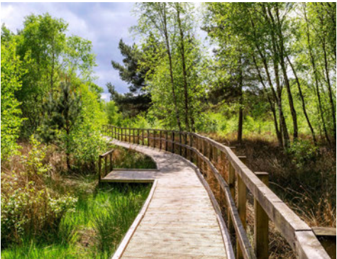
Timber boardwalk through wetland/heath
