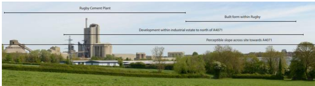
Figure 2: Views to the north-east towards industrial development and development within Rugby seen on higher ground
