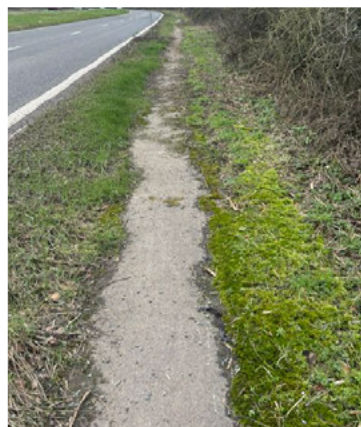
Photograph 3: Existing footway along A45
