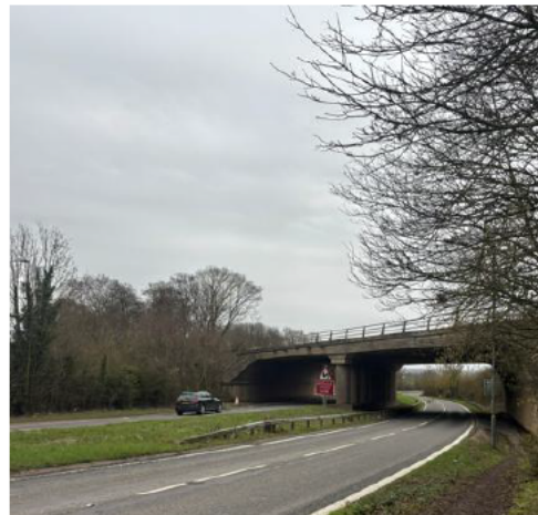
Photograph 2: A45 facing south
