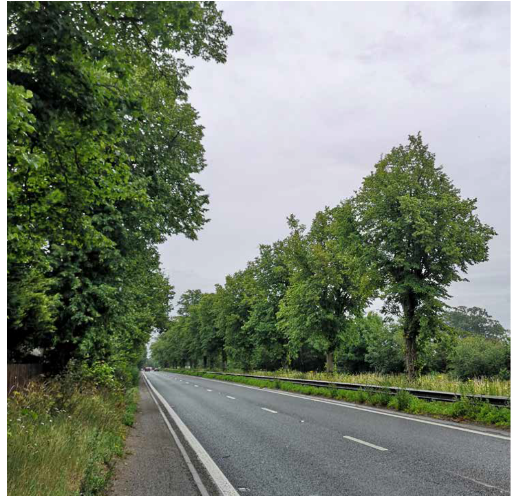
View along the A45 close to Stretton on Dunsmore exit
