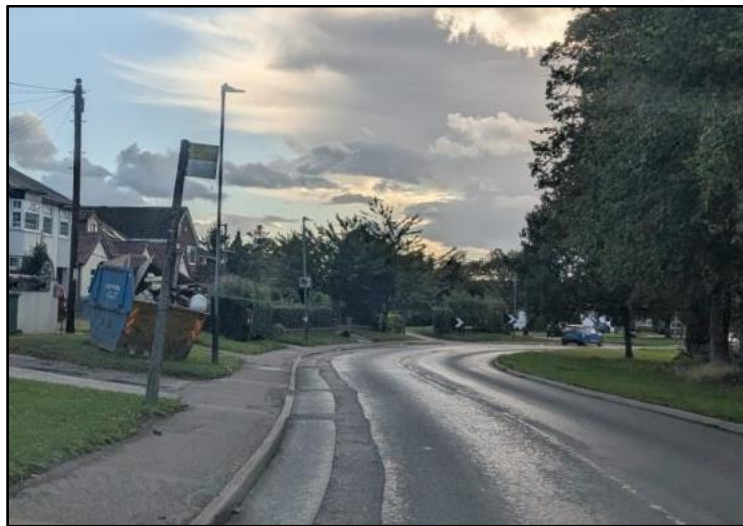
Figure 4 – Narrow Footways and Bus Stop on Rugby Road
