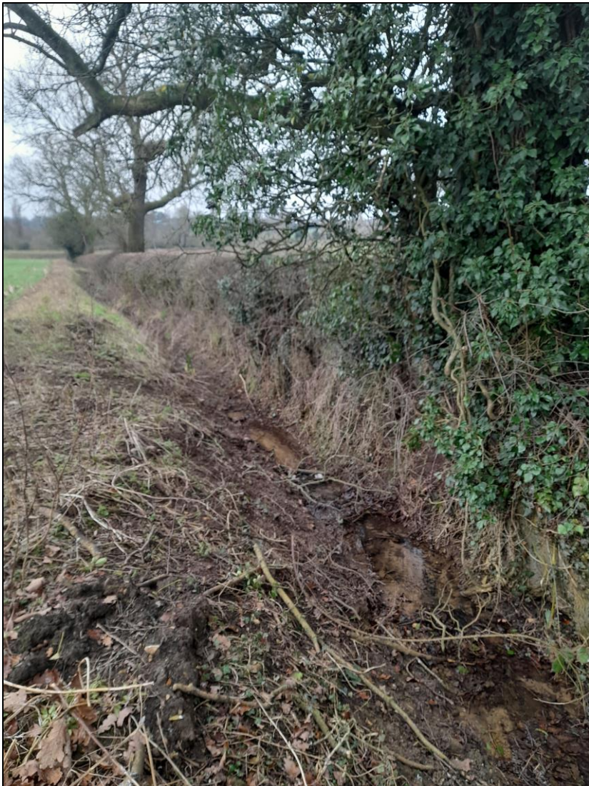
Figure 1: View from Culvert A (Pond Outfall) looking downstream
