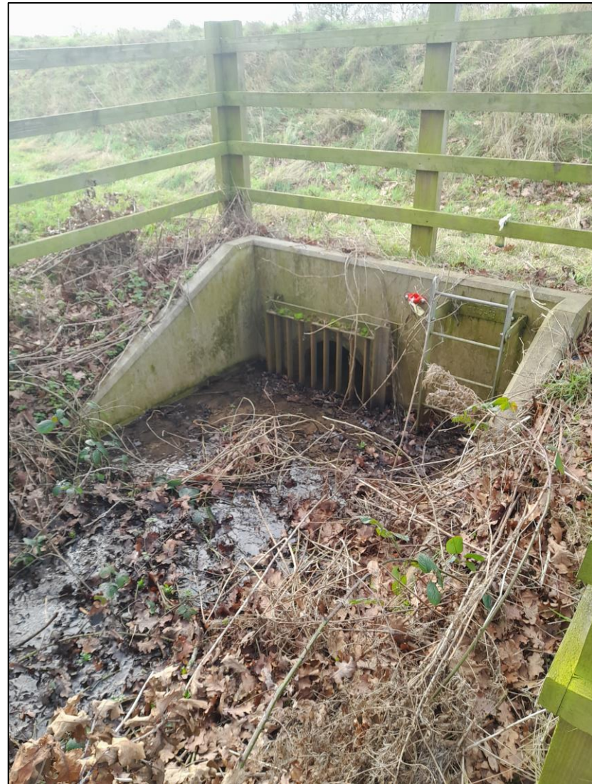
Figure 2: View towards Culvert C (Houlton Way) looking downstream
