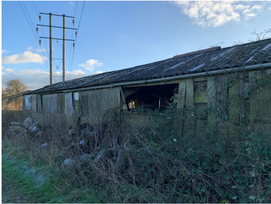
Photograph 2: showing the exterior of B1
