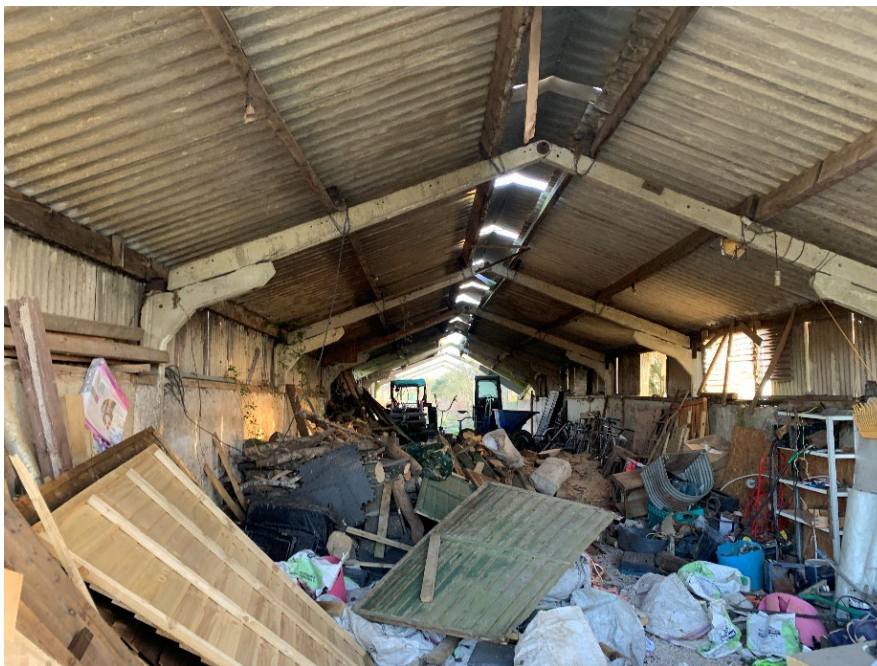
Photograph 1: Showing the interior of B1
