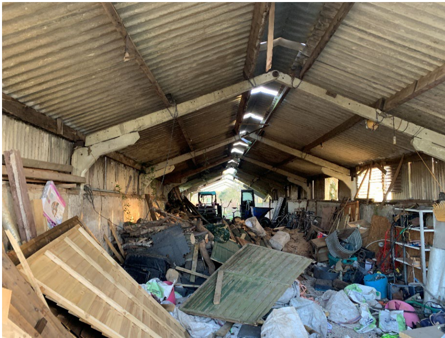
Photograph 1: Showing the interior of B1
