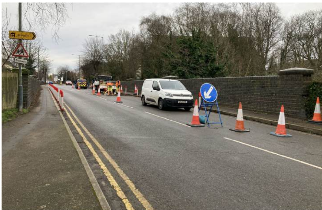
Figure 4-10 - Carriageway and footway surfacing from eastern side
