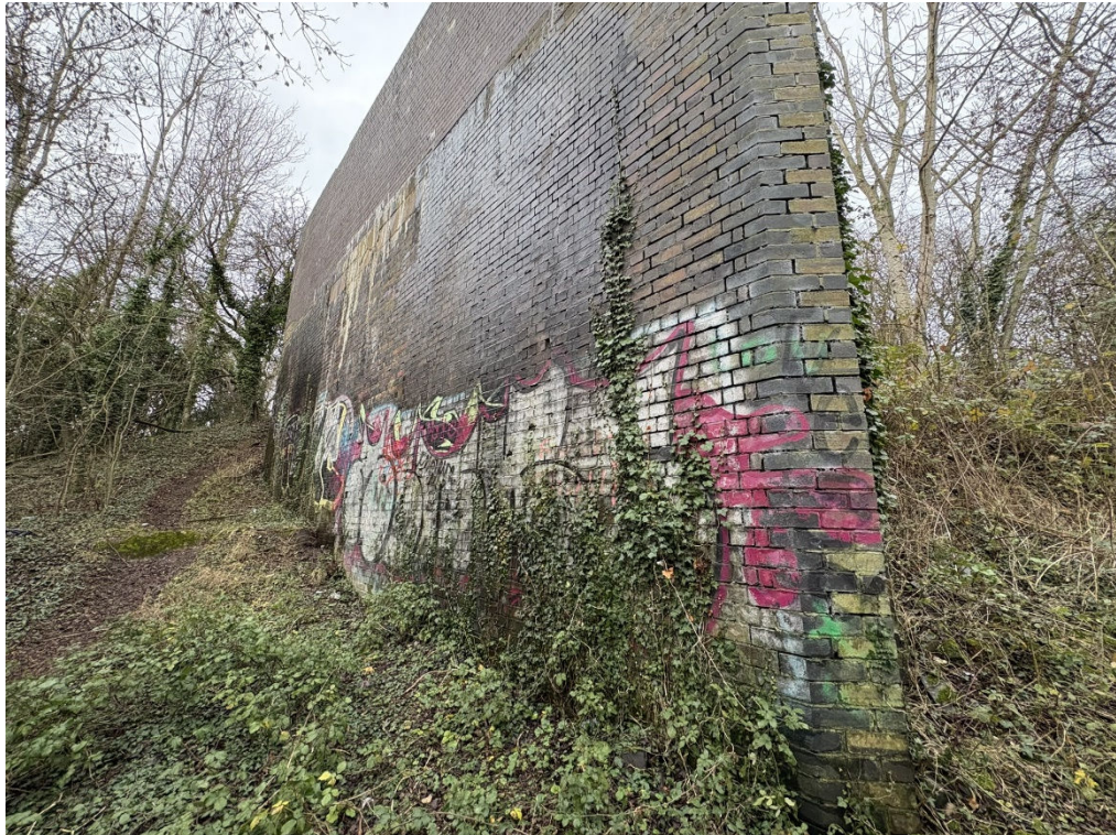
Photograph 1 General view of the front face of retaining wall, at the southeast corner, looking northwest.
