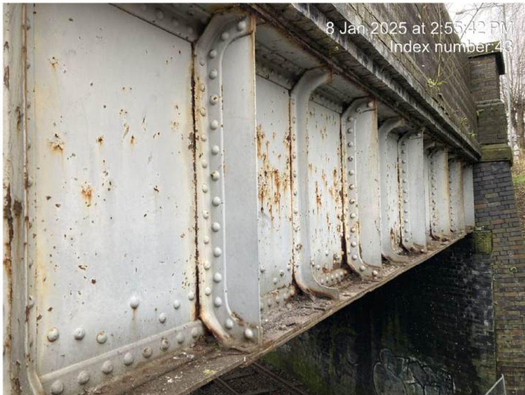
Figure 4-1 - Outer girder (north)
