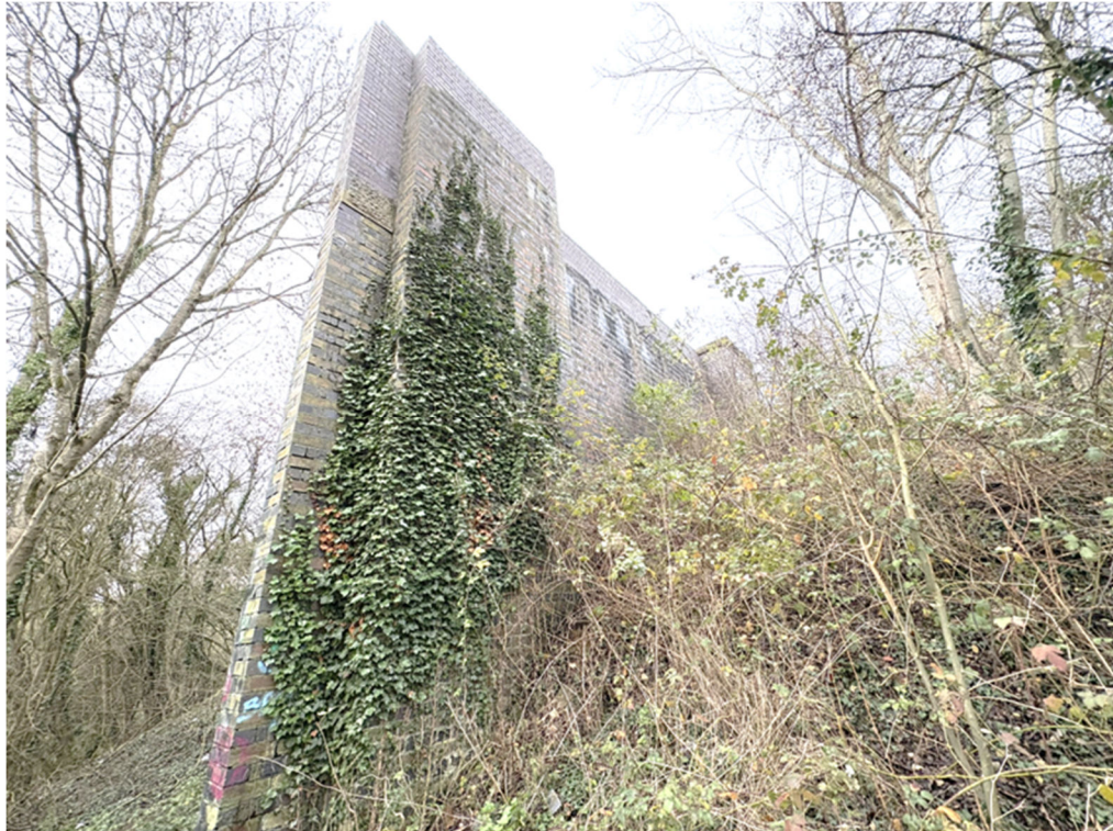
Photograph 2 General view of the east side face, looking west.
