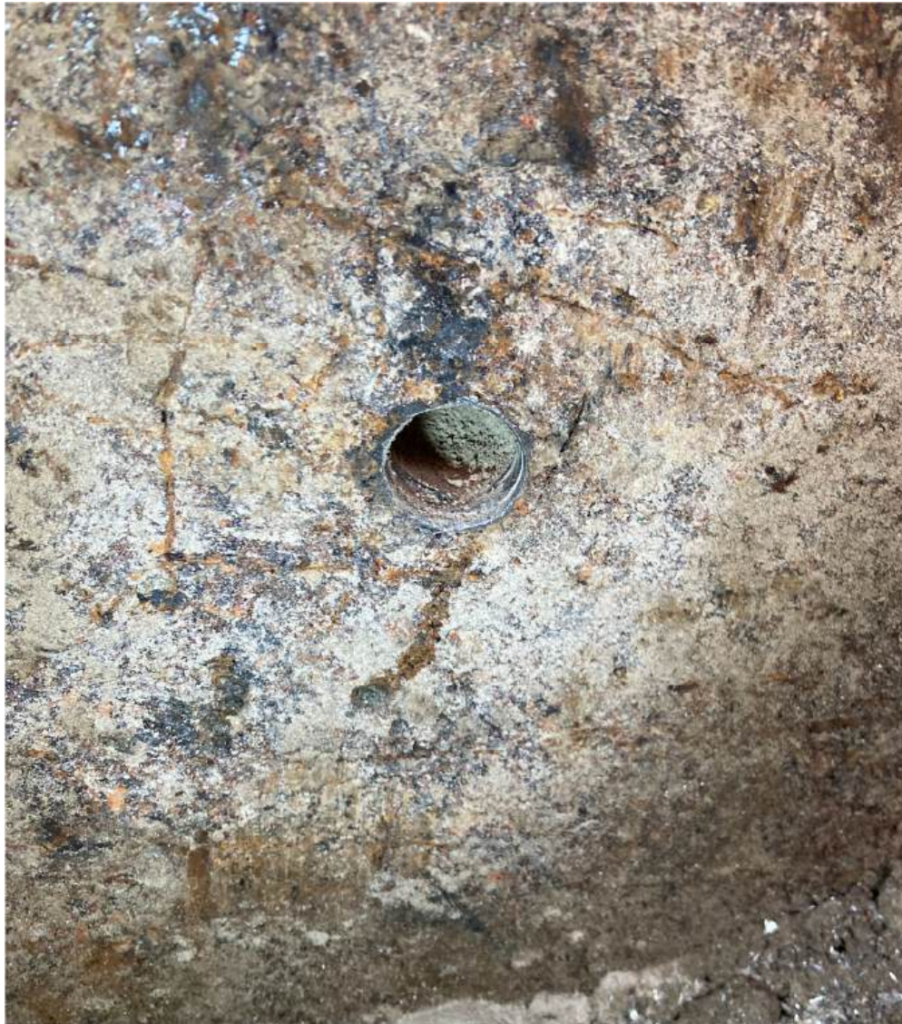
Figure 7-1 - Drilled hole in internal girder web
