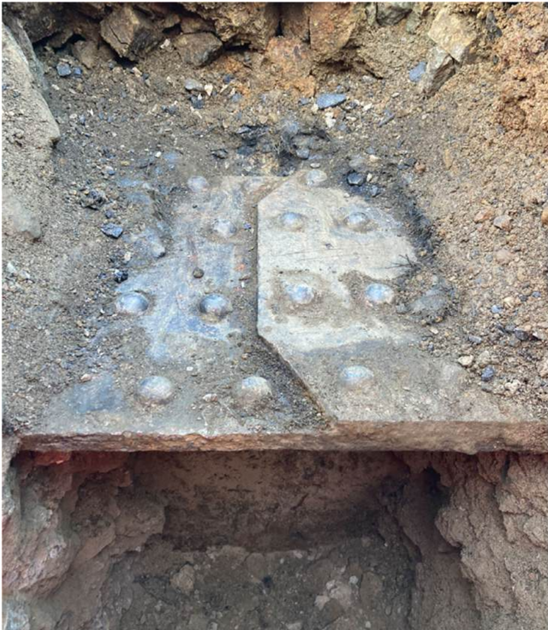
Figure 7-9 - Top flange of longitudinal girder in trial pit TP1
