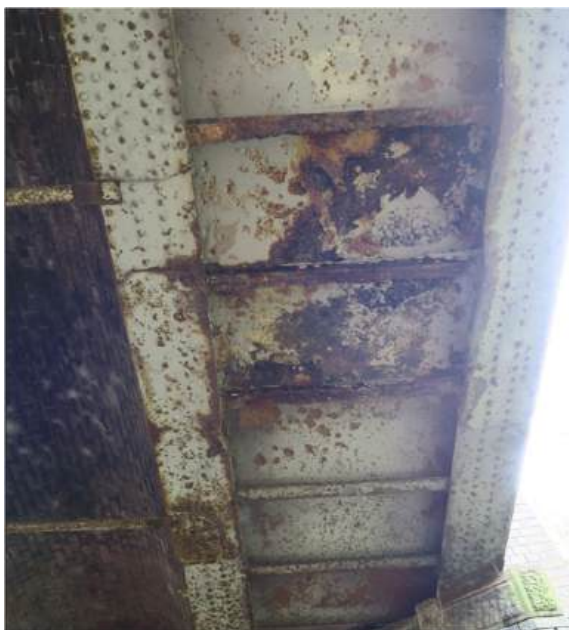
Figure 7-4 - Outer and inner girders with cover plate removed (NW)
