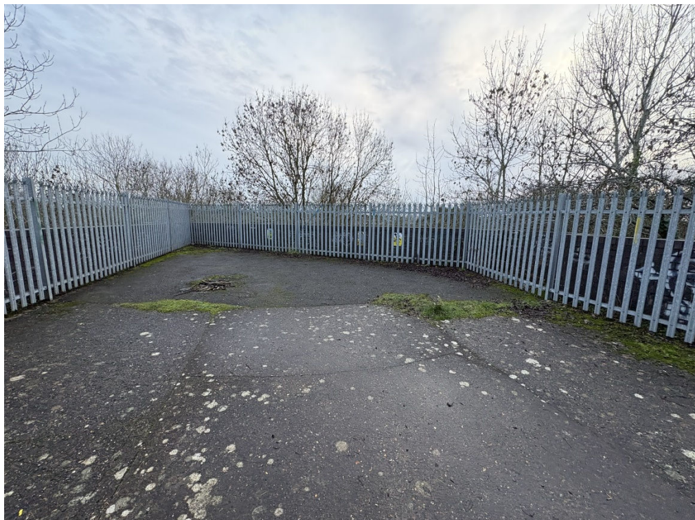
Photograph 4 General view of the topside of the wall, looking south.
