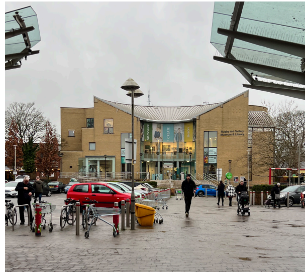
Main Northern Approach from Chapel Street
