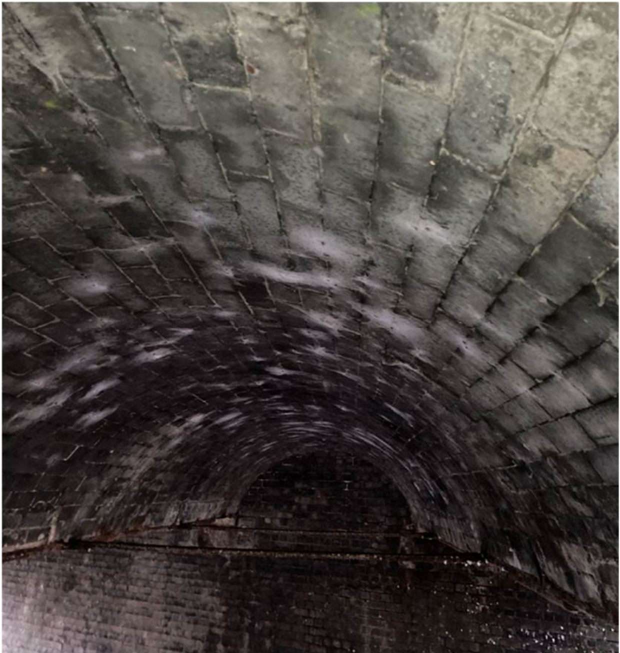
Figure 4-5 - View below typical transverse masonry arch
