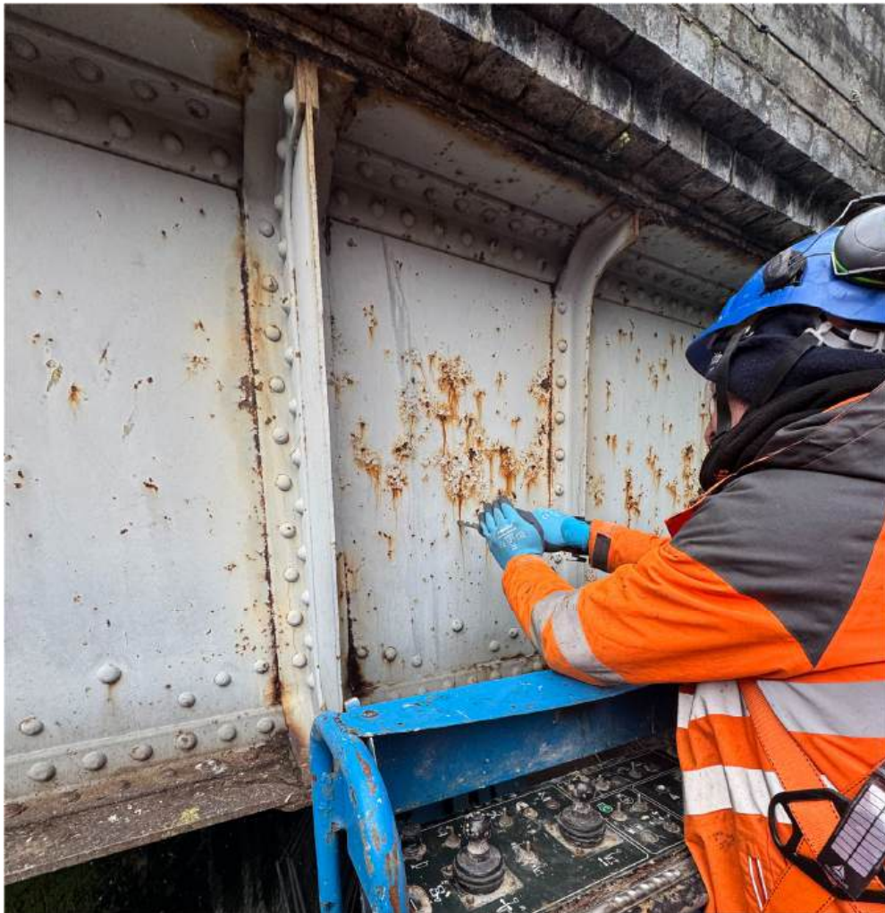
Figure 7-2 - Drilled hole in outer girder web on the south side
