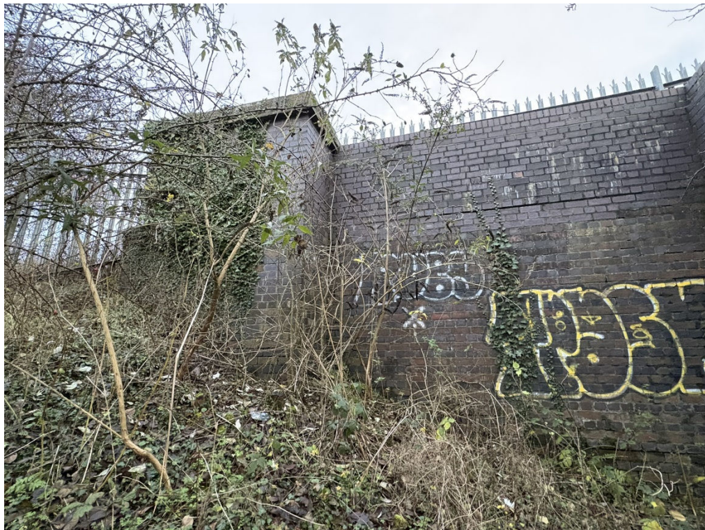
Photograph 3 General view of the west side face, looking east.
