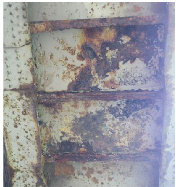
Figure 7-4 - Outer and inner girders with cover plate removed (NW)
