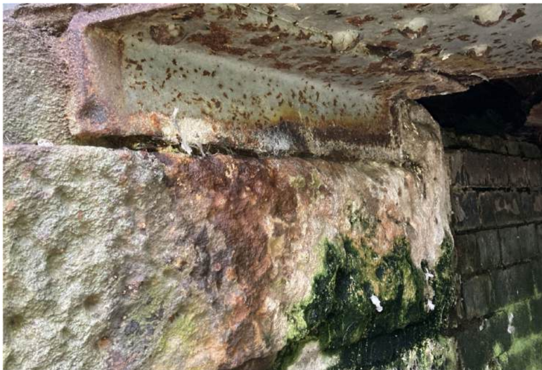
Figure 4-7 - Sandstone bearing plinth
