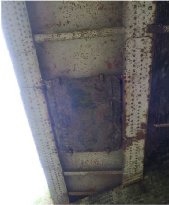
Figure 7-3 - Outer and inner girders and cover plate (NE)
