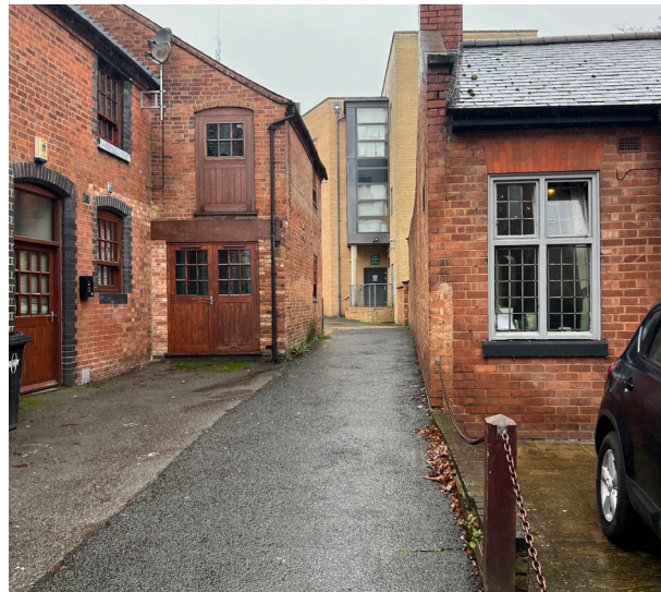
West Side Service Approach
