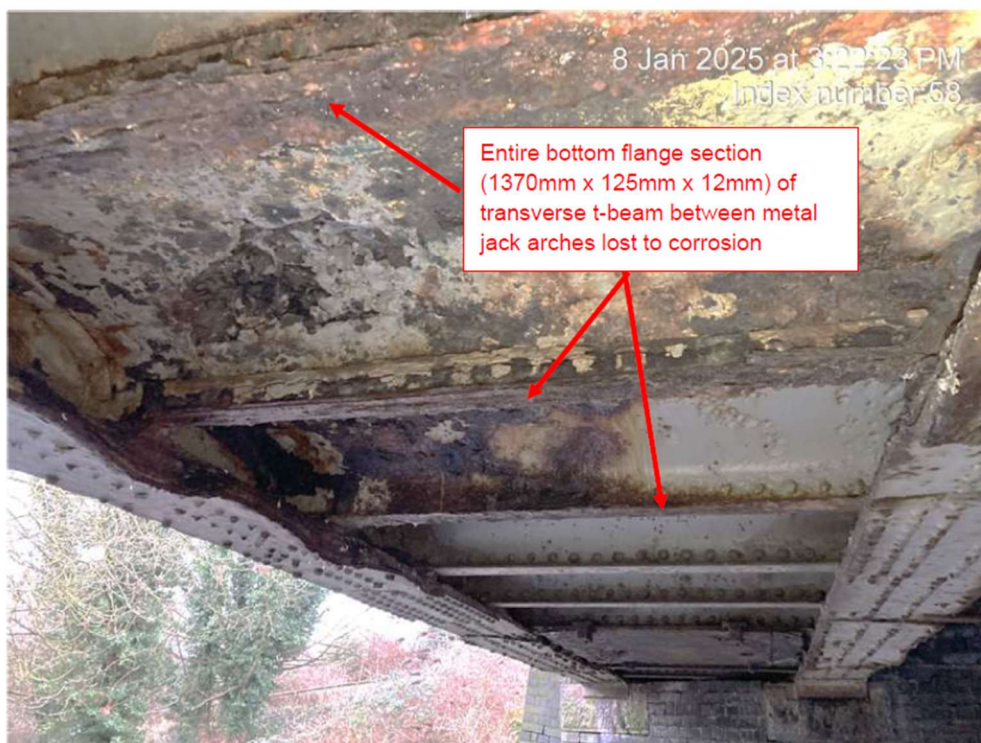
Figure 4-4 - Metal arches spanning longitudinally between 2 outermost girders
