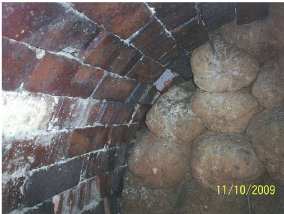
Figure 3: Concrete bag work at west end from inside of culvert from Scott Wilson Ltd Principal Inspection Report (2009)
