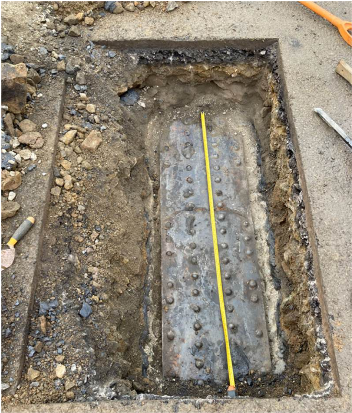
Figure 7-10 - Top flange of longitudinal girder in trial pit TP2
