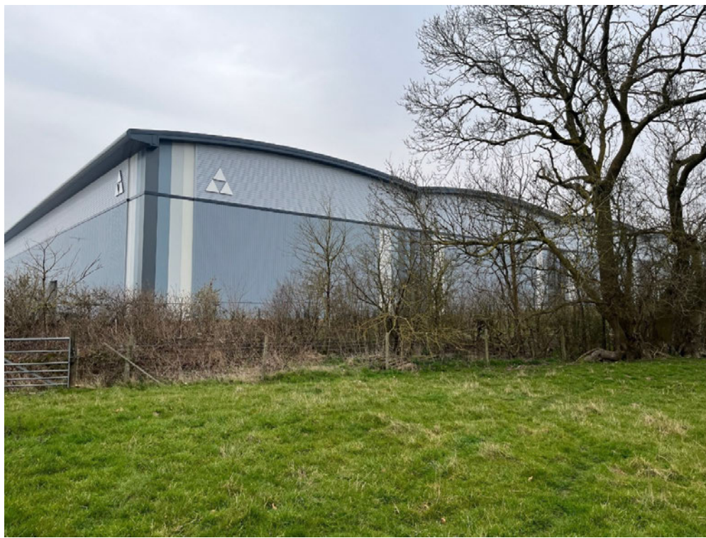
Photo 7 View to the North, of Tritax Warehousing
