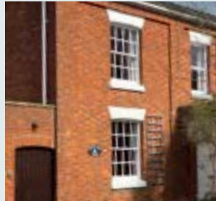
Sash window with glazing bars
