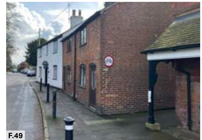
Figure 49: Terraced cottages along Lilbourne Road within the village core.
