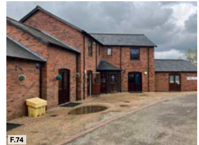
F.74 Figure 74: Office building frontage with small courtyard area for parking.
