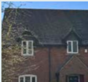
Gable dormer windows
