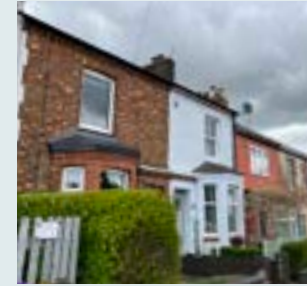
Mix of red brick and colour finishes
