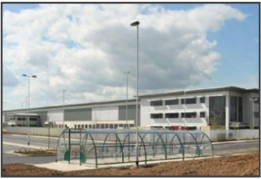
Enhanced facade system to meet air tightness as low as 1.5m3/hr/m2 at 50Pa
