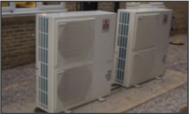
Air Source Heat Pumps to provide low carbon heating & cooling
