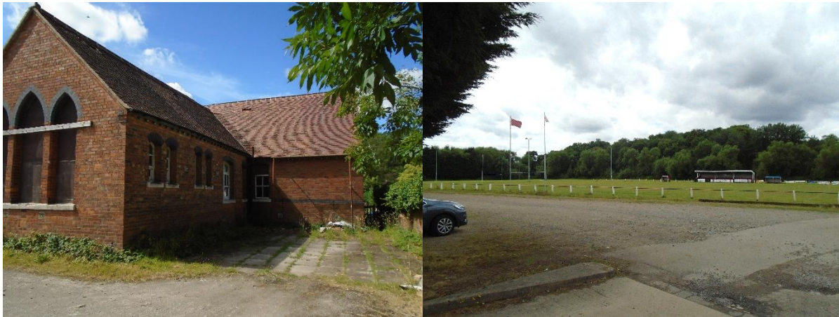
Left: View of the rear of Newbold Village Hall showing slipped roof tiles, faulty rainwater goods and boarded windows. Right: The extensive grounds of Newbold on Avon Rugby Football Club.
