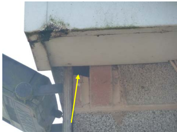
Building 3 - typical access points for bats at soffit and fascia
